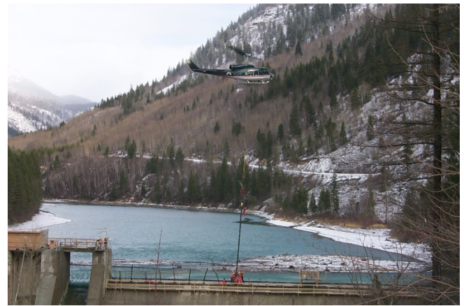
Installation of a post-tensioned anchor in the spillway
