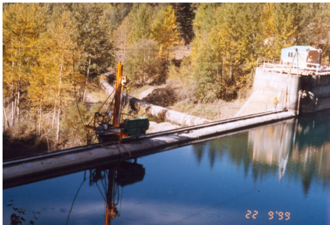
Drilling holes for the post-tensioned anchors
