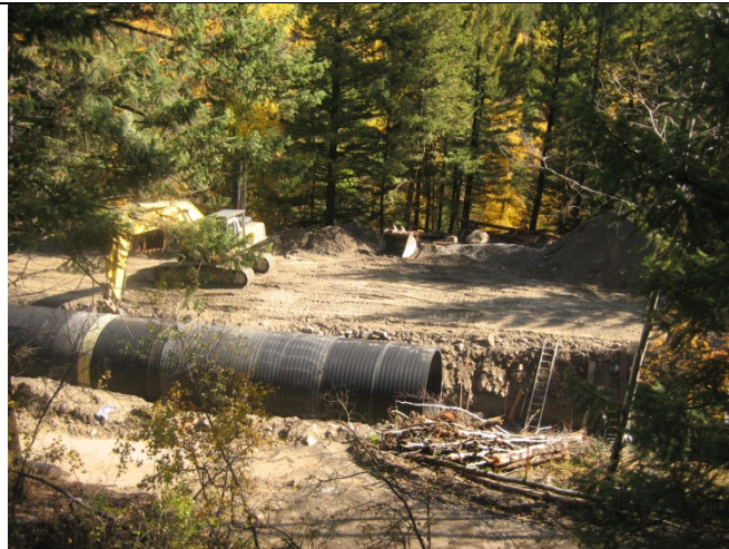
Construction of the new penstock
