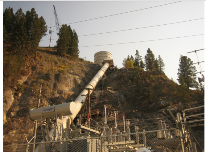
New steel penstock and surge tower
