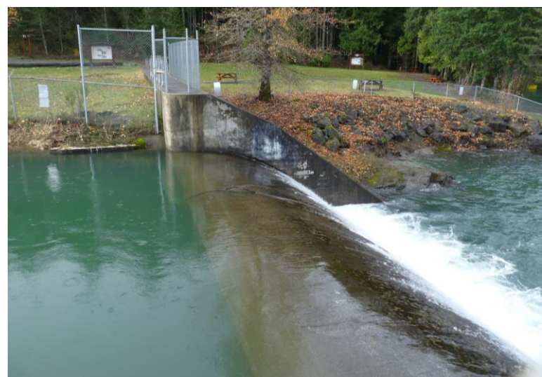
Photo 3 – Spilling over the Free Overflow Spillway
