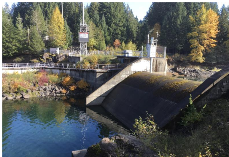
Photo 2 – Free Overflow Spillway with Fishway in background
