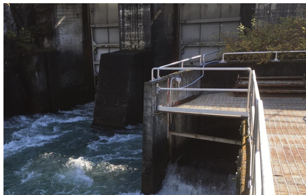
Photo 4 – Downstream face of Sluice Gates and Fishway
