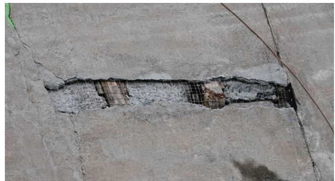
Figure 15 Large repair area chipped open and exposed on the face of La Joie Dam during this year's annual maintenance.
