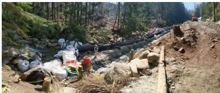
Figure 6 Water diversion in place at Boulder Creek and rip rap placement occurring at the dyke toe.
