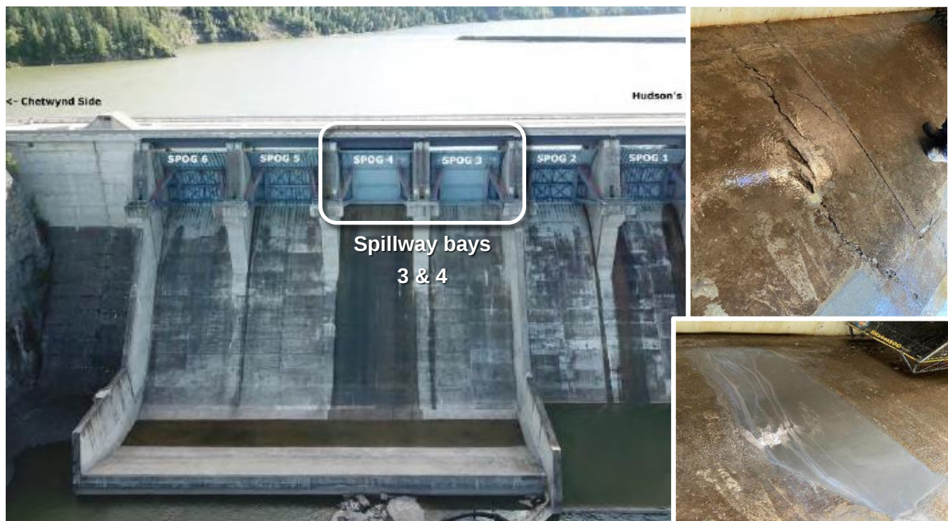
Figure 7 Peace Canyon Dam spillway concrete repairs: (Left) Location of repairs; (Upper right) crack in bay 3 between stoplog and spillway gate sills; (Lower right) repaired crack.
