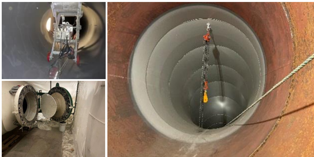
Figure 9 Recoating of the Bridge River 2 Penstock 2. Top left: coating robot inside the penstock. Bottom left: New access hatch installed by the project. Right: penstock before (foreground) and after (background) recoating.
