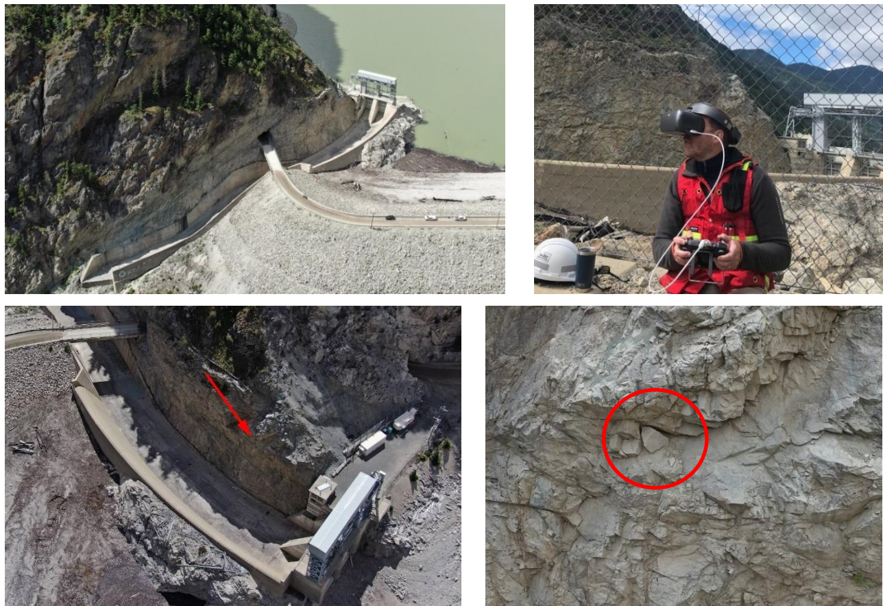
Figure 11 Terzaghi Dam spillway chute rock wall inspection. Overview (top left), engineer controlling the drone's high resolution camera (top right), location of a loose, hazardous rock (bottom left), and close-up view of the hazardous rock which is approximately 0.6 metres or 2 feet wide (bottom right).
