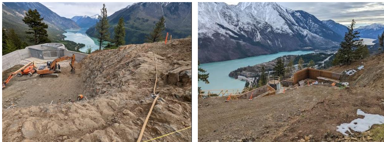
Figure 8 Construction of the containment basins at the top of the east (left) and west (right) surge shafts at the Bridge River 1 Generating Station.
