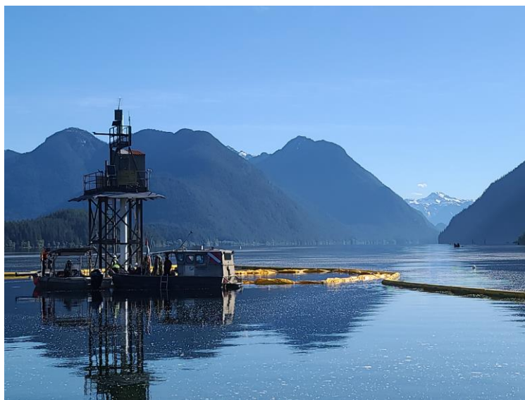
Figure 5 Alouette Dam low level intake with dredging underway.
