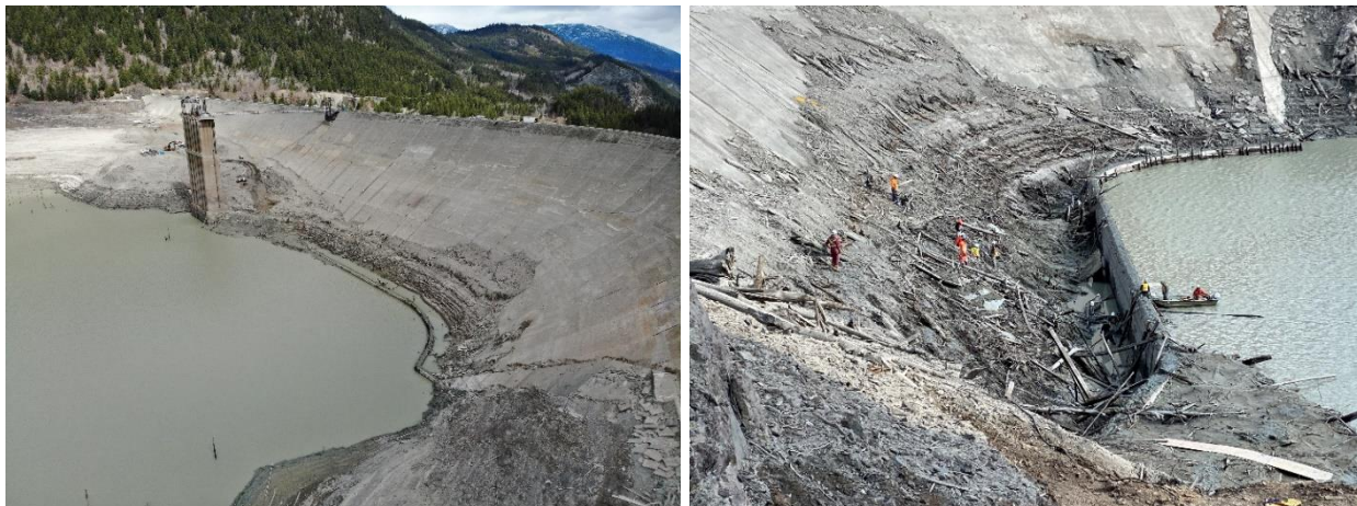
Figure 10 La Joie Dam during the spring 2022 drawdown. Note the significant volume of debris located on the toe of the dam.
