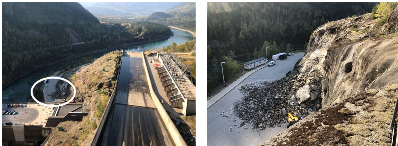
Figure 3 Rockfall on the Marble Shear Block at Revelstoke Dam and Generating Station. At left: the location of the rockfall as viewed from above the spillway. At right: view of the rockfall onto the access road and main parking lot of the generating station.
