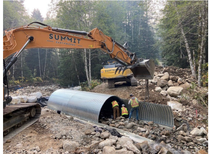
Figure 8 Installation of a new culvert under the Wahleach Dam access road to prevent future washout.
