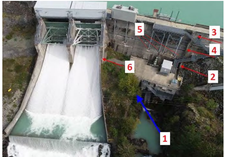
Figure 4 Drone photo showing areas of Cheakamus Dam where concrete is deteriorating due to alkali aggregate reactivity.
