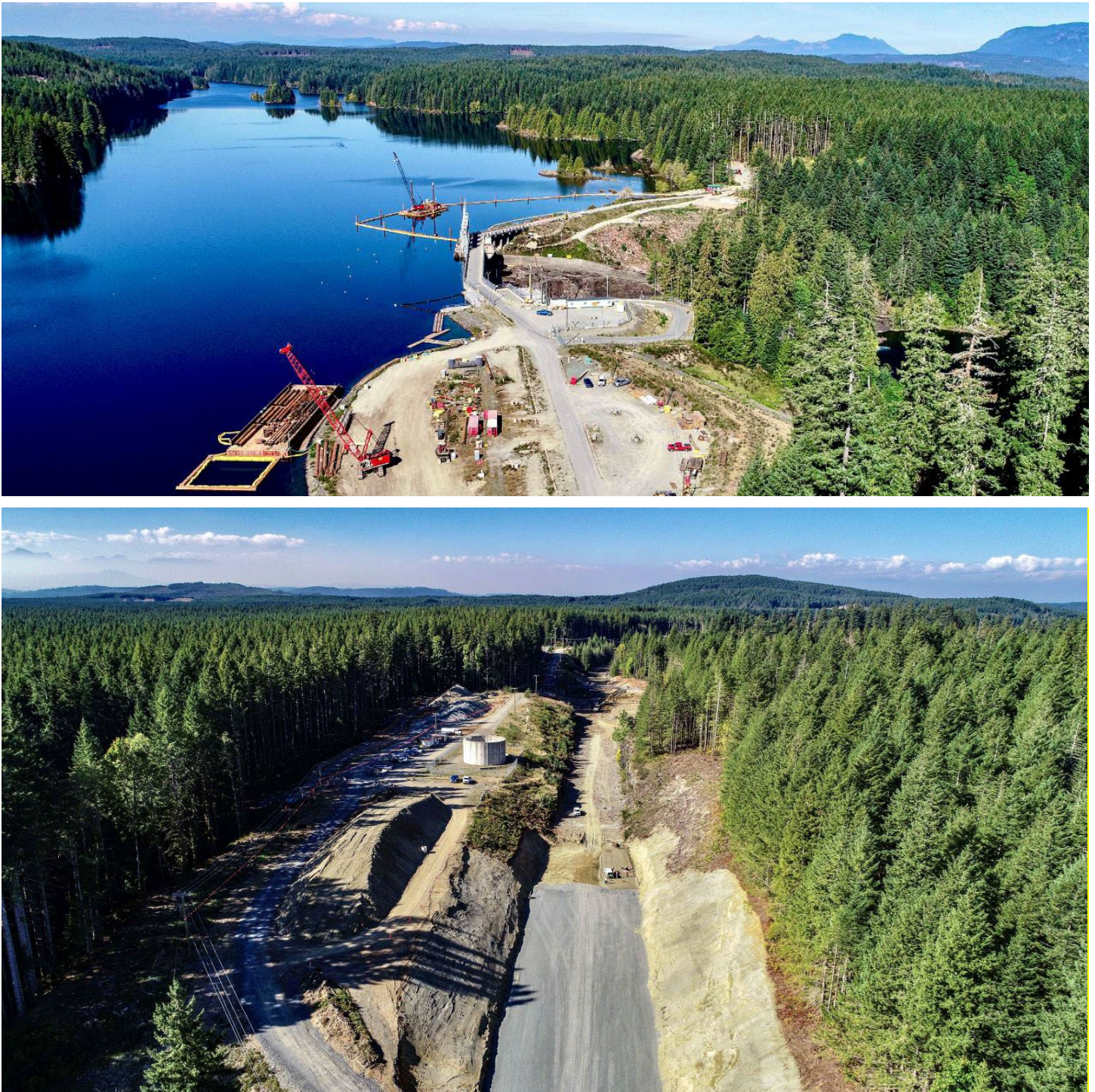
Figure 9 Construction on the John Hart Dam Seismic Upgrade Project is underway, as seen in these September 8 photos from the site. Top: Work area on the Middle Earthfill Dam (foreground) and installation of the silt curtain upstream of the North Earthfill Dam (background). Bottom: Construction of one of three containment berms along the old penstock corridor, where dredgeate from the reservoir will be placed.
