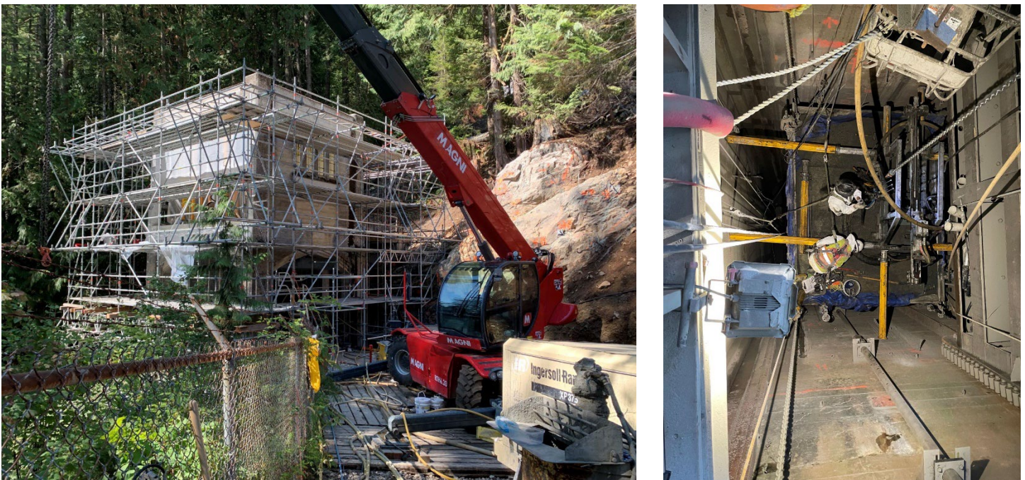
Figure 7 Seismic upgrades underway on the structures of the Alouette Tunnel. At left: surge tower superstructure. At right: surge shaft concrete lining; work being performed from suspended platform that is raised and lowered along the shaft as required.
