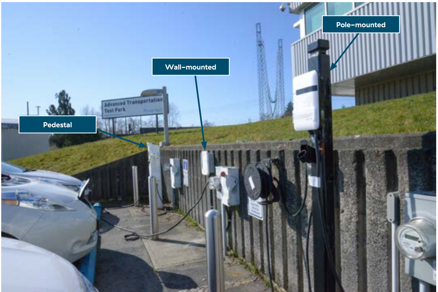
FIGURE 4. NOSED IN CHARGING STATION AND VARIOUS LEVEL 2 CHARGER INSTALLATION.
