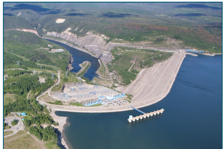
Gordon M. Shrum Generating Station & W.A.C. Bennett Dam
