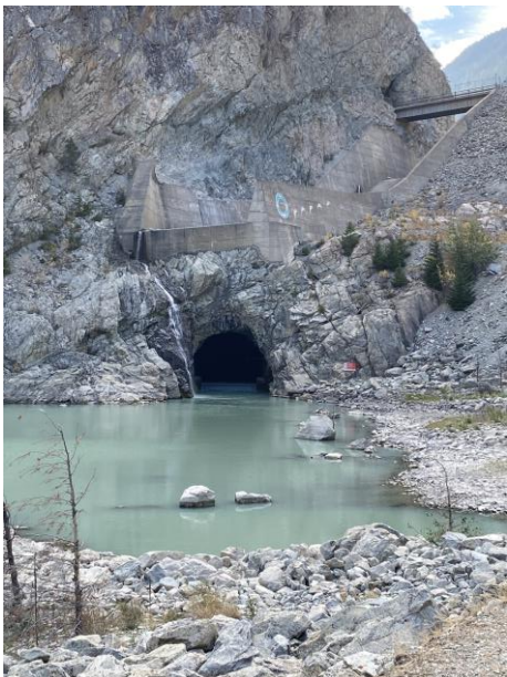
Terzaghi spillway and low-level discharge outlet
